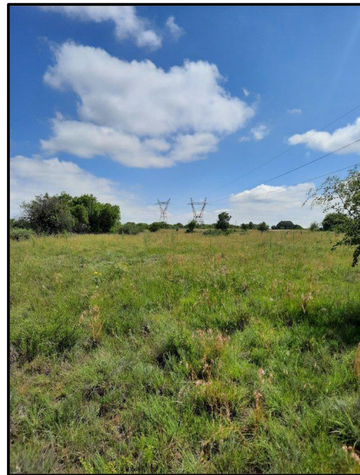
Figure 5.4. Powerline in the study area.
