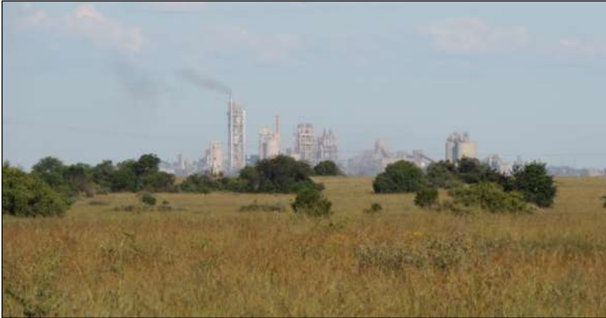
Figure 7. Zoomed photograph of the Lichtenburg LaFarge Cement Factory that forms a background view to the development areas.
