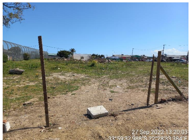
Fig.2: View west at site entry/exit point off Golf Street. Note partially demolished building in centre of site.
