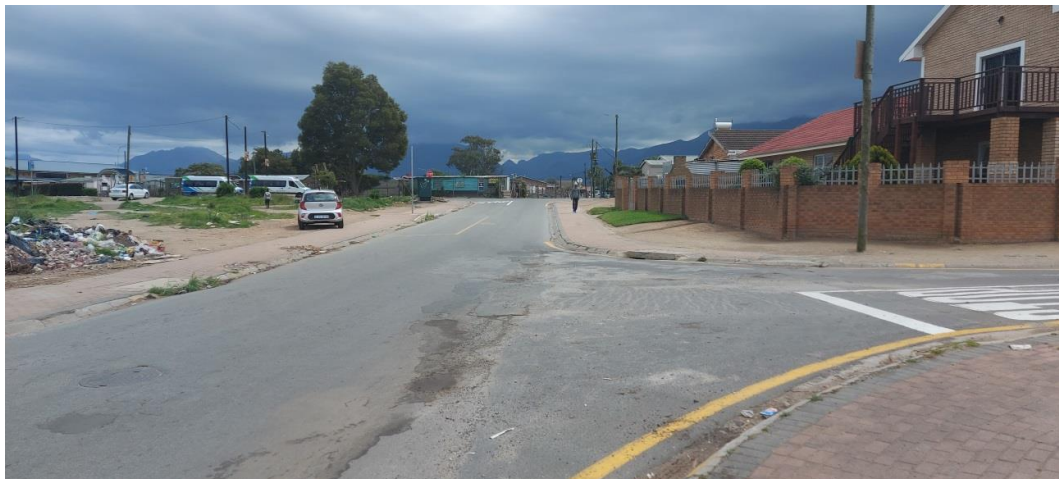
Existing sidewalks along Golf Street
