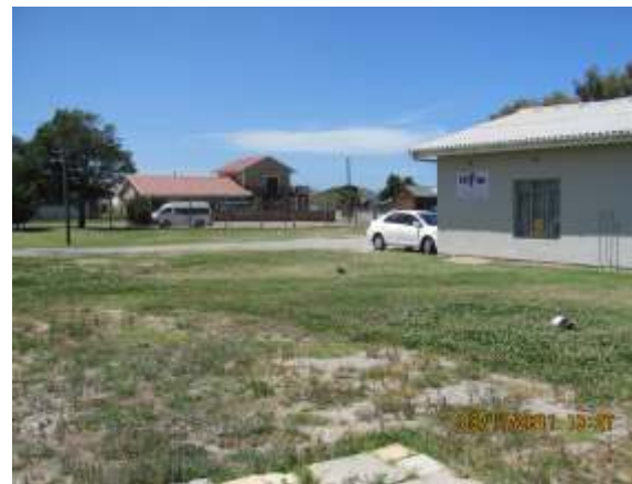
Photo 4-6: Existing infrastructure on Erf 11221
