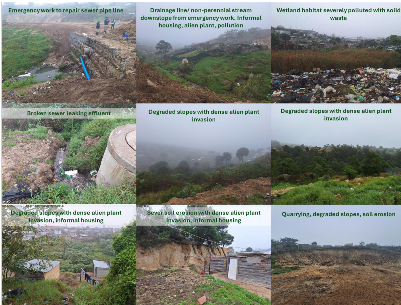
Figure 10. Site photos depicting prolific negative impacts and transformed habitats within the Thembalethu sewer line project area.
