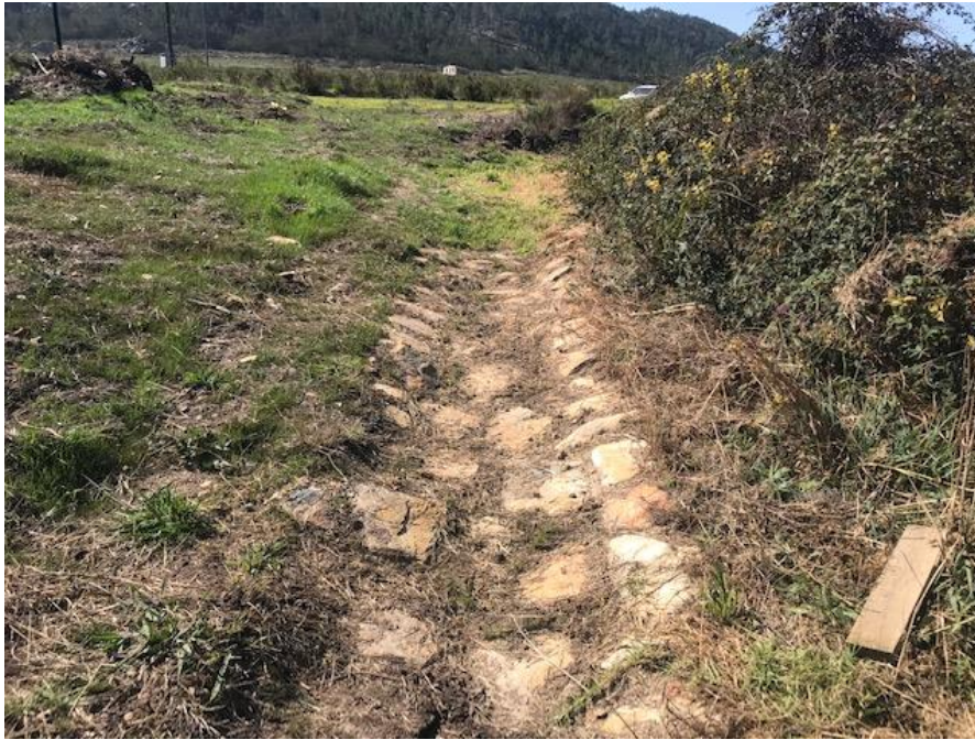
Figure 14. Example of a simple spillway, grassed on low gradient and protected with natural rock in earth on steeper slope. Vegetation has been mowed, but leaving vegetation like grass to grow between stones will provide additional protection.
