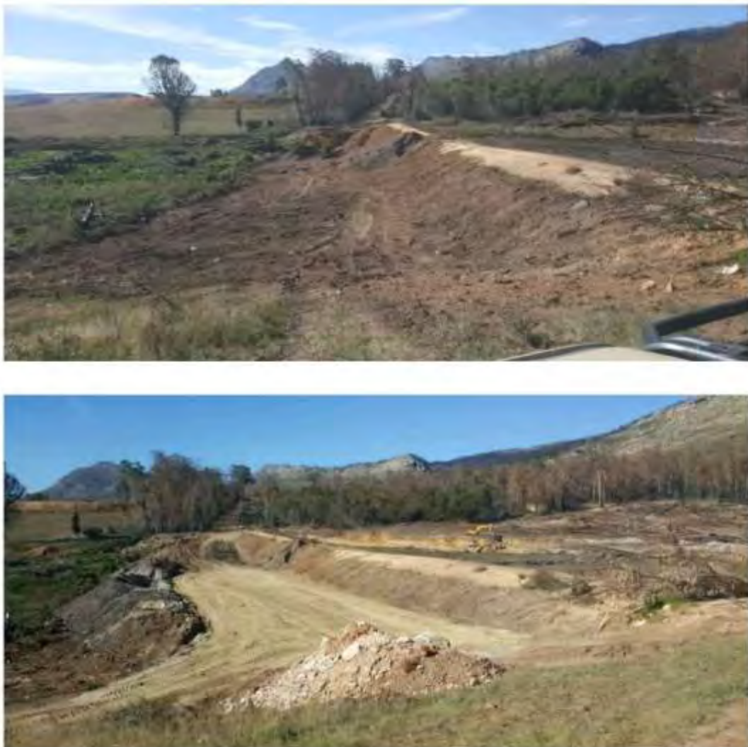
Figure 1: Images taken during construction showing the widening of the existing dam wall to strengthen and seal it, as well as excavation of silt from the dam basin.
