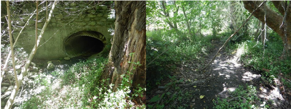
Figure 4: Photographs illustrating the watercourse to the south of the development footprint.
