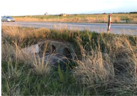
Inlet of culvert draining underneath R102
