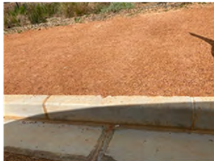
Stabilised gravel sidewalk surfacing
