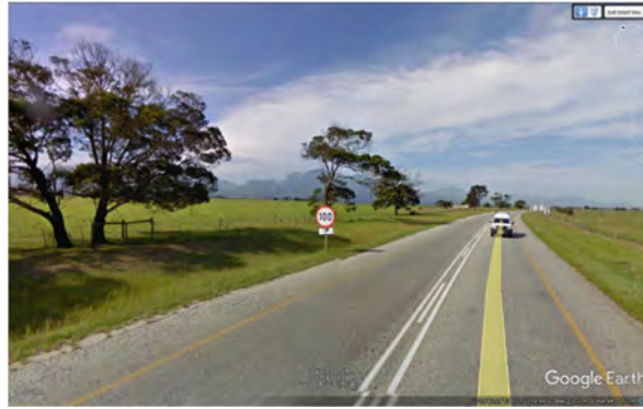
Side drains on both sides of R102
