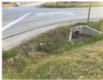
Culvert inlet draining from east to west under R404
