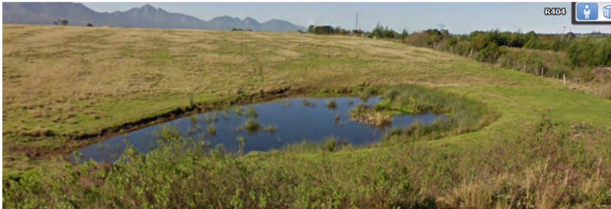
Stormwater dam on Erf 1 of Portion 4
