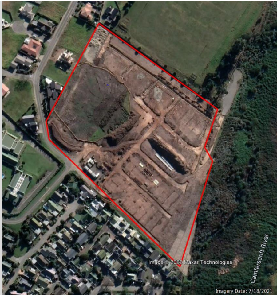
Figure 2: Google image showing earthworks with platforms and internal road works.
