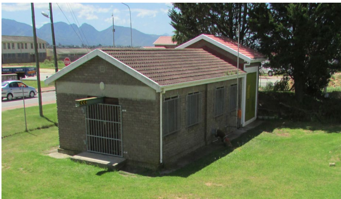
Figure 7: Existing pumpstation PWT-PS-01
