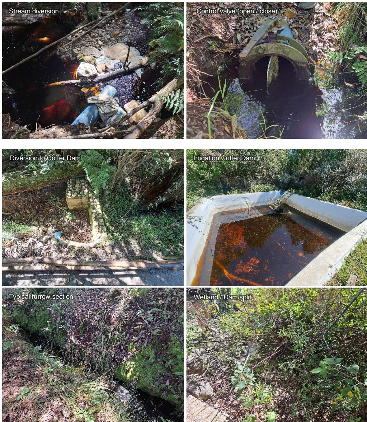
Figure 10. Photos of key operational points and features along the furrow supplying water to the botanical gardens dam mapped in Figure 9.
