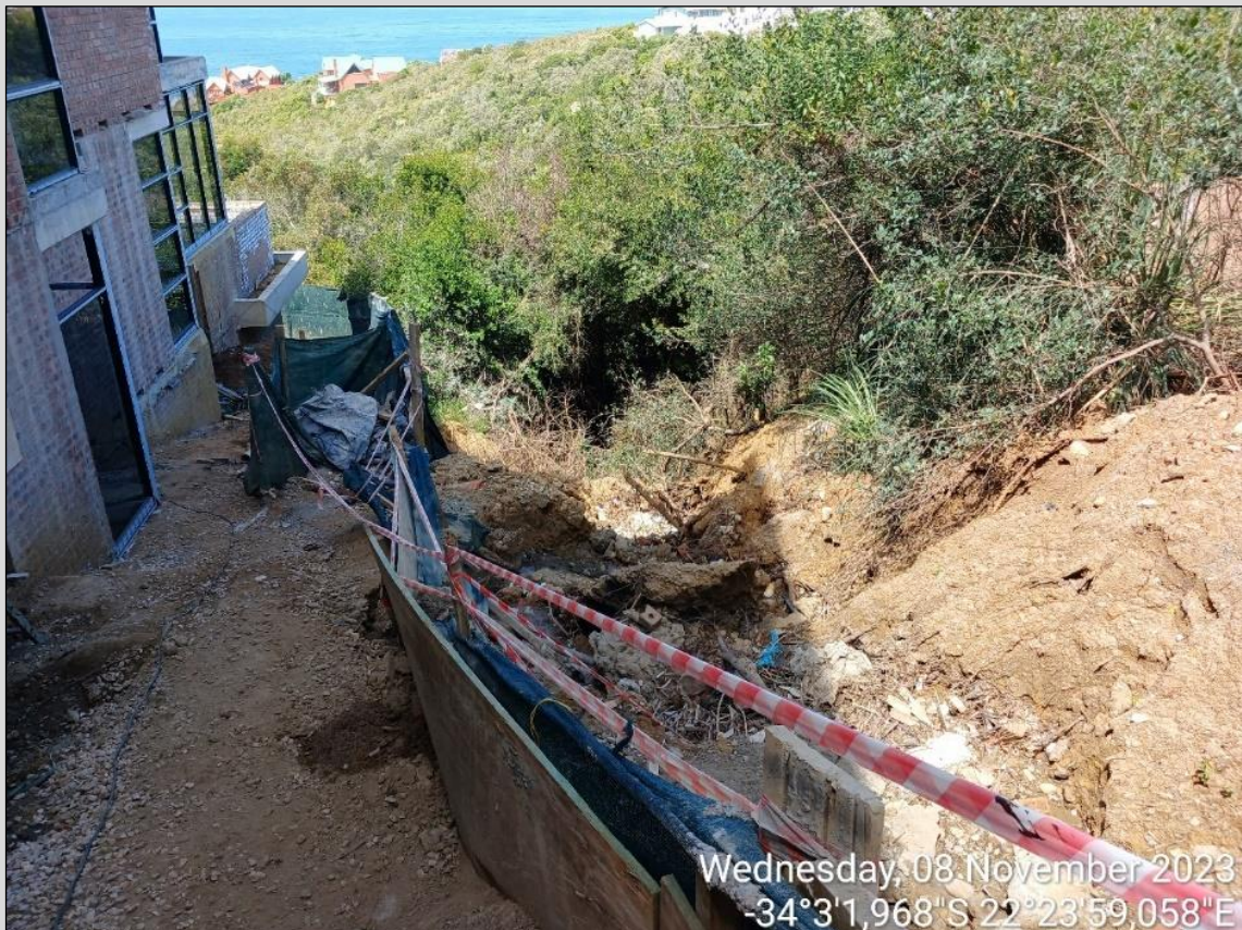
Figure 4: Photograph of Erf 318. This area has been disturbed through a combination of stormwater runoff and what appears to be constructed related activities on Erf 318 where building rubble have been dumped into the erosion gully.
