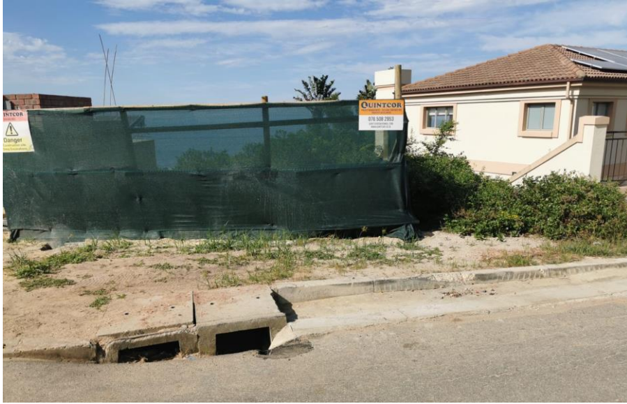
Fig. 4: The location of Erf 318 (located behind the green shade cloth screen), between one developed property (on the right) and a property that is under construction (to the left). The section behind the screen is eroding rapidly, and needs to be stabilised as soon as possible.
