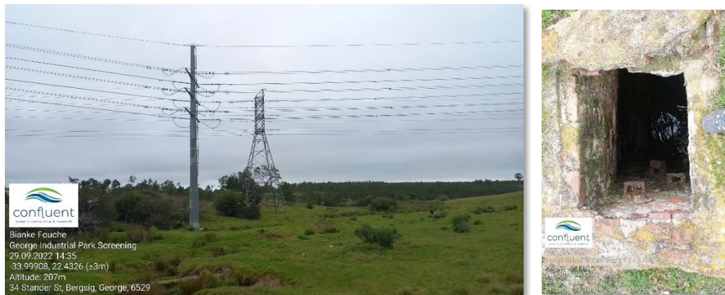
Figure 27: Left - an image of the power lines on the site, and the disturbed habitat below. Right – a hazardous open drain on the site
