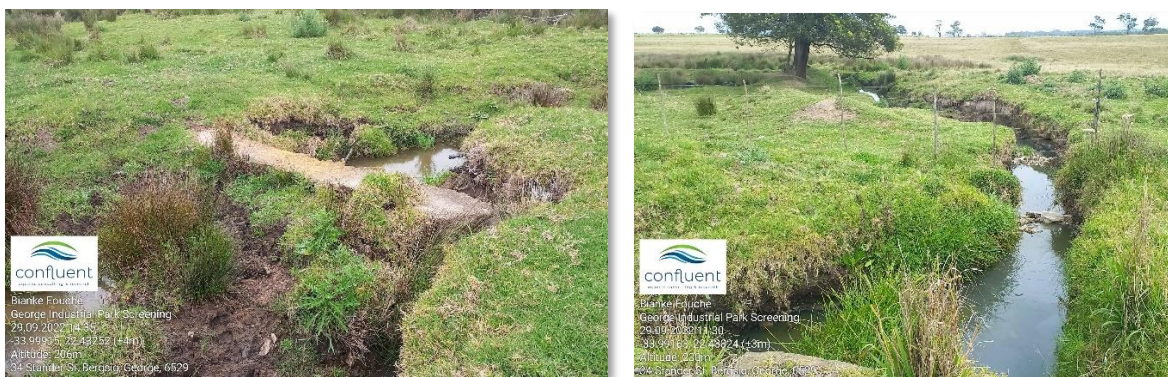
Figure 28: Left – Erosion around a cement weir. Right – steep eroded channel sides, with a black wattle tree standing on the bank.
