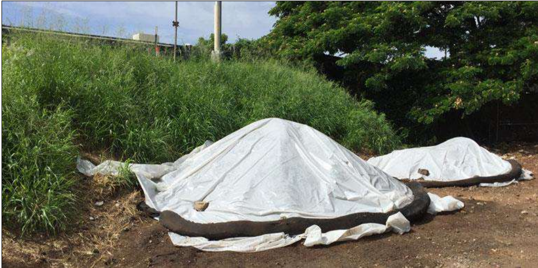
Figure 21: Stockpiles of fine textured building materials and soils covered with geotextile/plastic covering and banded with sandbags when not in use.
