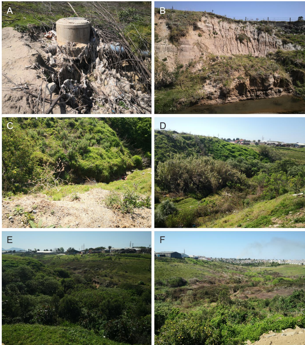
Figure 12: A – Leaking sewer infrastructure 10 m 10 m east of the Skaapkop River, B – Skaapkop River with eroding banks on the West, C – General vegetation present at HGM1 with the channel of HGM1 filled with building rubble, D – CVB at the lower reach of HGM1, E – CBV at the confluence of HGM1 and HGM2 looking in a north-westerly direction, F – CBV at the confluence of HGM2 and the Skaapkop River looking in a southern direction.
