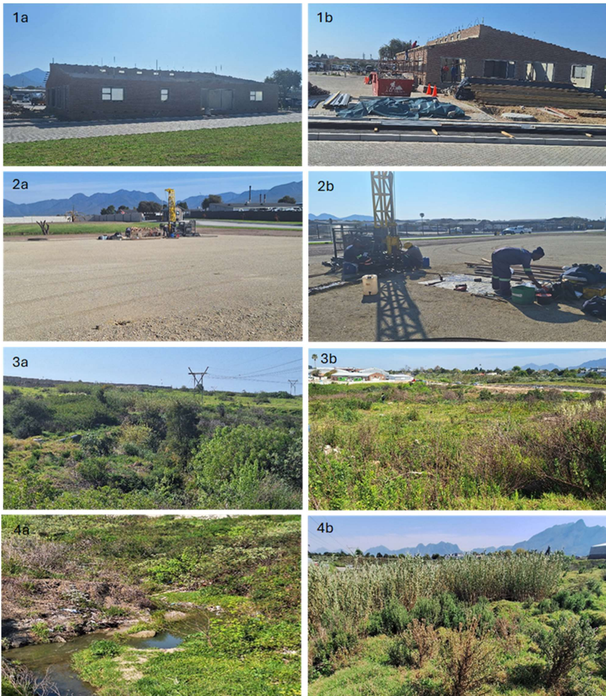
Figure 10: Images from the site inspection conducted at the George Municipal Depot, ErF 464: (1a&b) Ongoing construction of new office building; (2a&b) Cleared area and ongoing activities on site where the new water depot is to be constructed; (3a&b) Area where future development is to occur ; (4a&b) Non-perennial river and artificial wetland in area where future development is to occur
