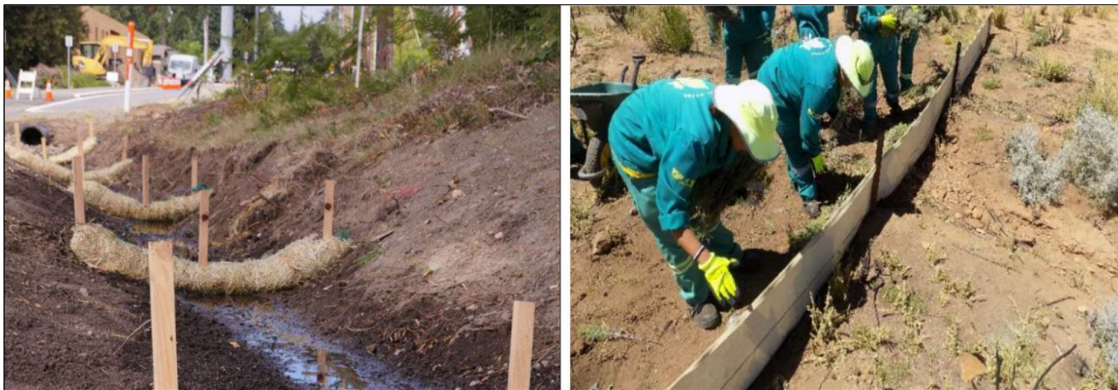
Figure 17. Examples of silt socks (left) and a silt fence (right) placed perpendicular to the flow of water. These methods reduce the force of water flow, erosion and can prevent unwanted sedimentation at the site.
