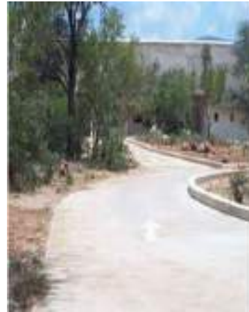
Figure 7 Completed cement surfaced road built with Hyson Cells
