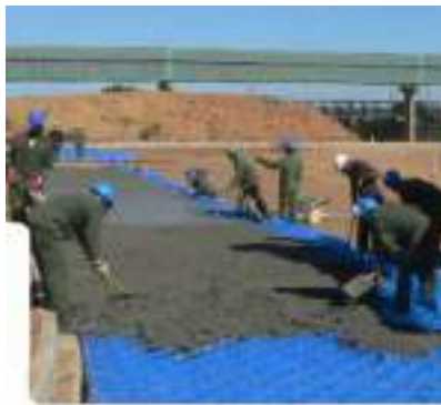
Figure 5 Hyson Cells filled with concrete
