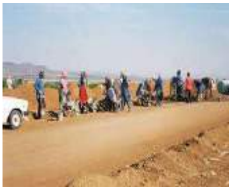
Figure 6 Gravel road built with Hyson Cells.
