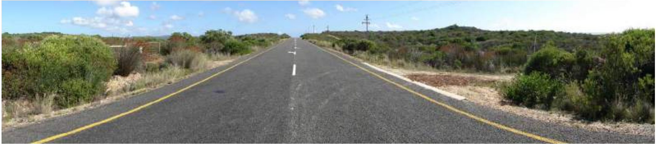
Photo 7: Northwest facing view along R325 (i.e. travelling from Gouritz towards N2). Access to lower-lying (eastern) portion of the property noted to right; access to higher-lying (western) portion of the property evident to the left.
