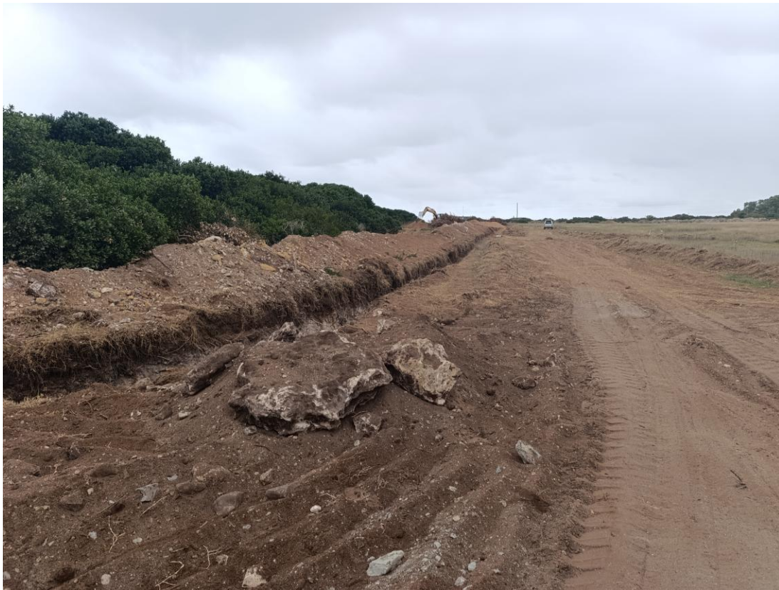
Photo 2: Construction along Phase 3 no-go areas, where the ECO was not provided with the opportunity to confirm correct demarcation before construction continued (photo taken 25 Feb 2025)
