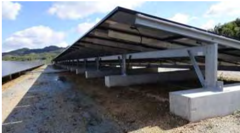
Figure 6: Cast Concrete Foundation (Solar Power Plant Business, 2013)
