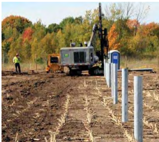
Figure 7: Driven/Rammed Steel Pile (SolarPro, 2010)
