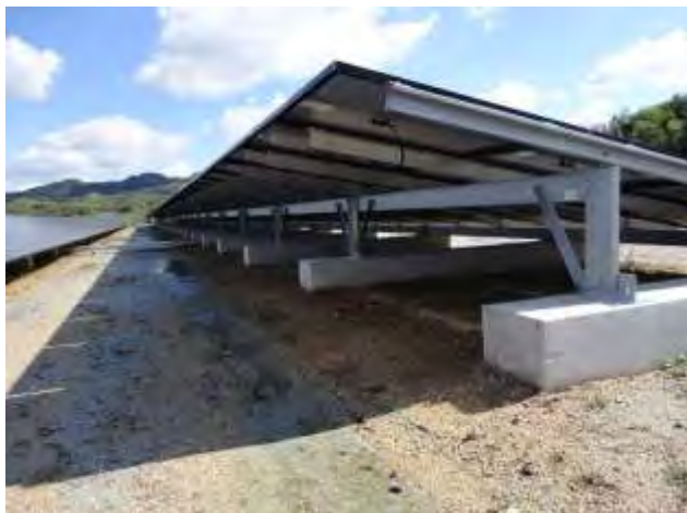
Figure 3: Cast Concrete Foundation (Solar Power Plant Business, 2013)
