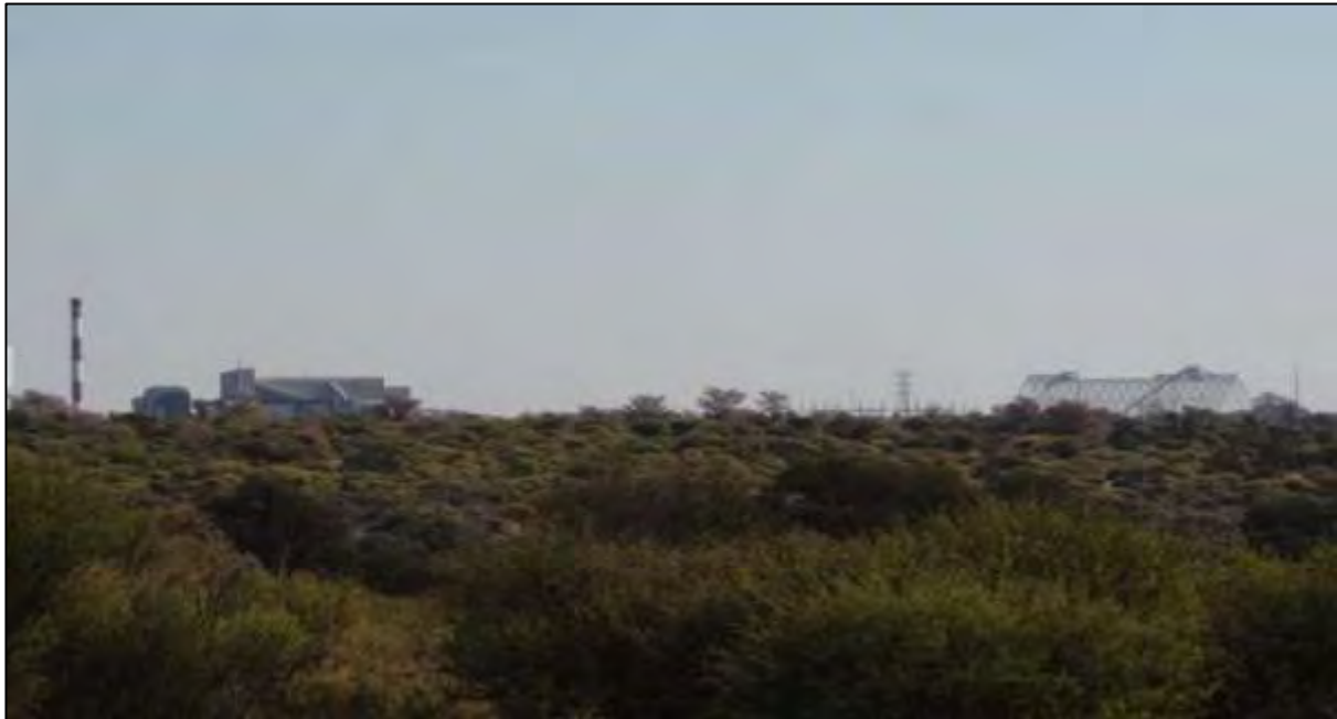
Figure 39: Photograph of the Kalagadi Manganese Mine as seen from the mine access road.
