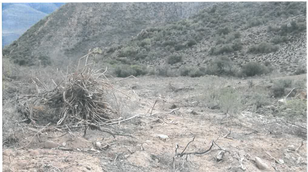
Photo 3: View of the destruction of vegetation cleared and topsoil disturbance within a watercourse with the construction of the new dam on the property.
