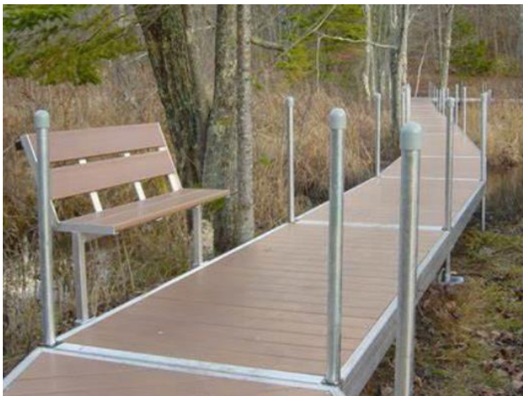
Figure 44: Example of modular lightweight boardwalk design allowing sections to be removed.
