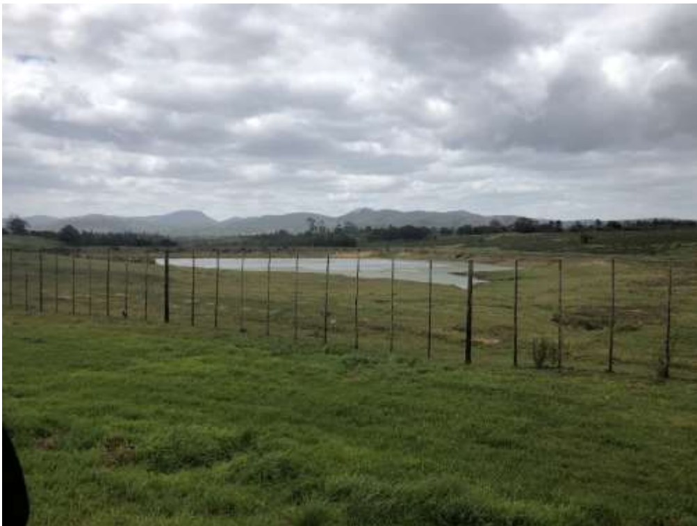
Plate 2: The approved water supply dam with no distinct aquatic habitat other than the open water itself
