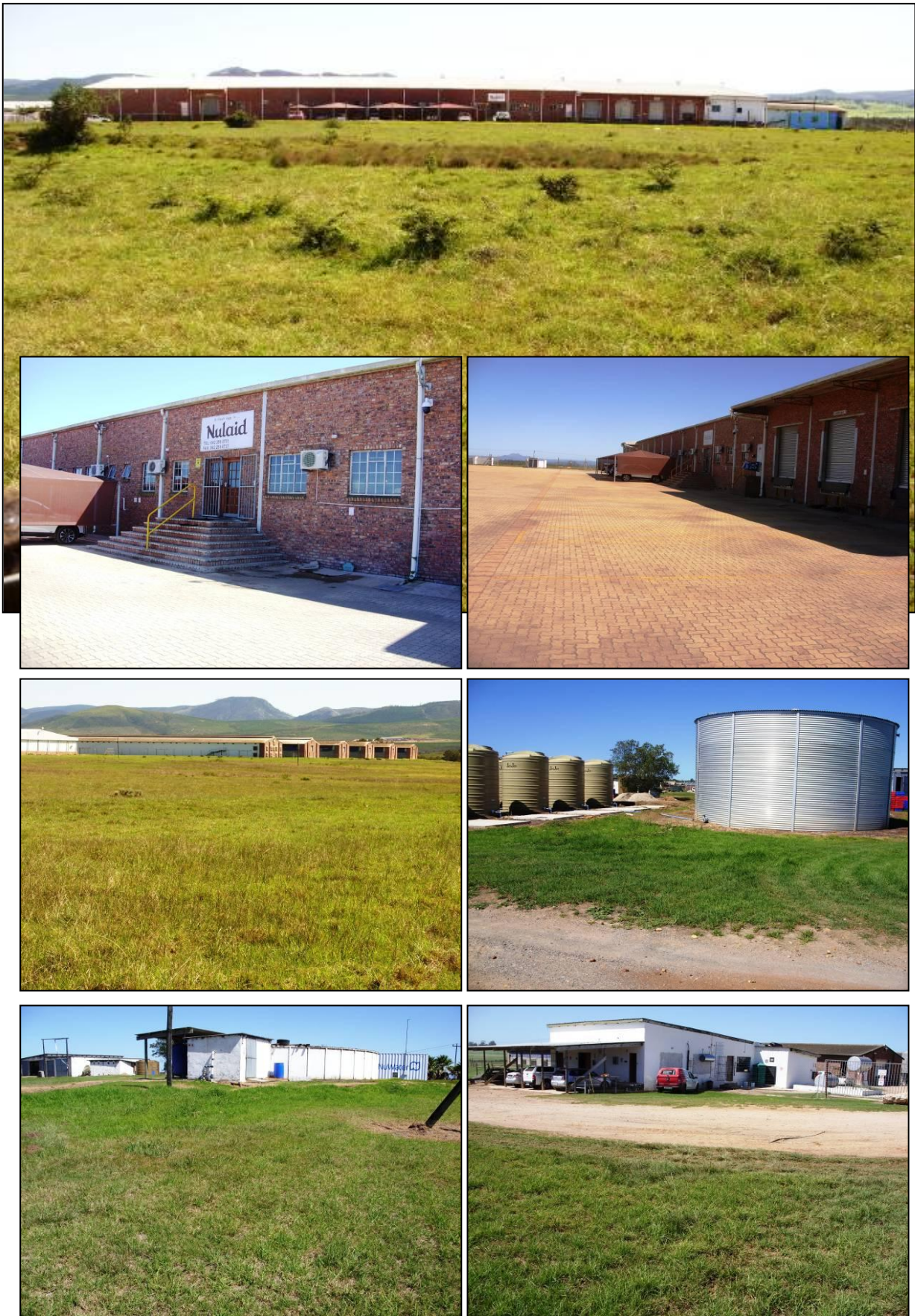
Figure 1. general views of the Quantum Foods egg laying facility near Thornhill.
