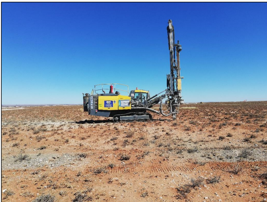
Figure 7: Pre-drilling of holes prior to the ramming of steel piles.
