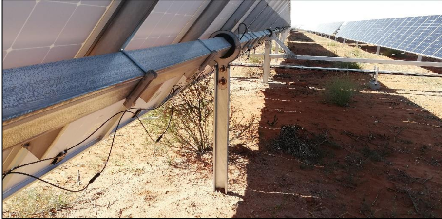
Figure 10: Completed racking and assembly showing vegetation remaining intact beneath the modules.
