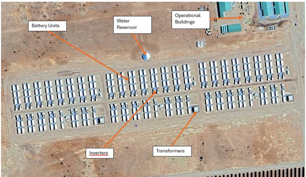
Figure 4: Typical configuration of a Solid-State Lithium BESS (Google Earth Image, 2024).
