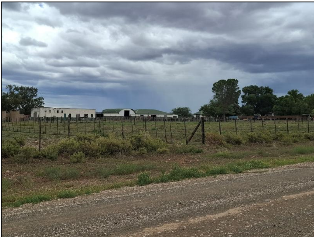
Photograph 3.14: Farmhouse complex on Bergrivier Farm
