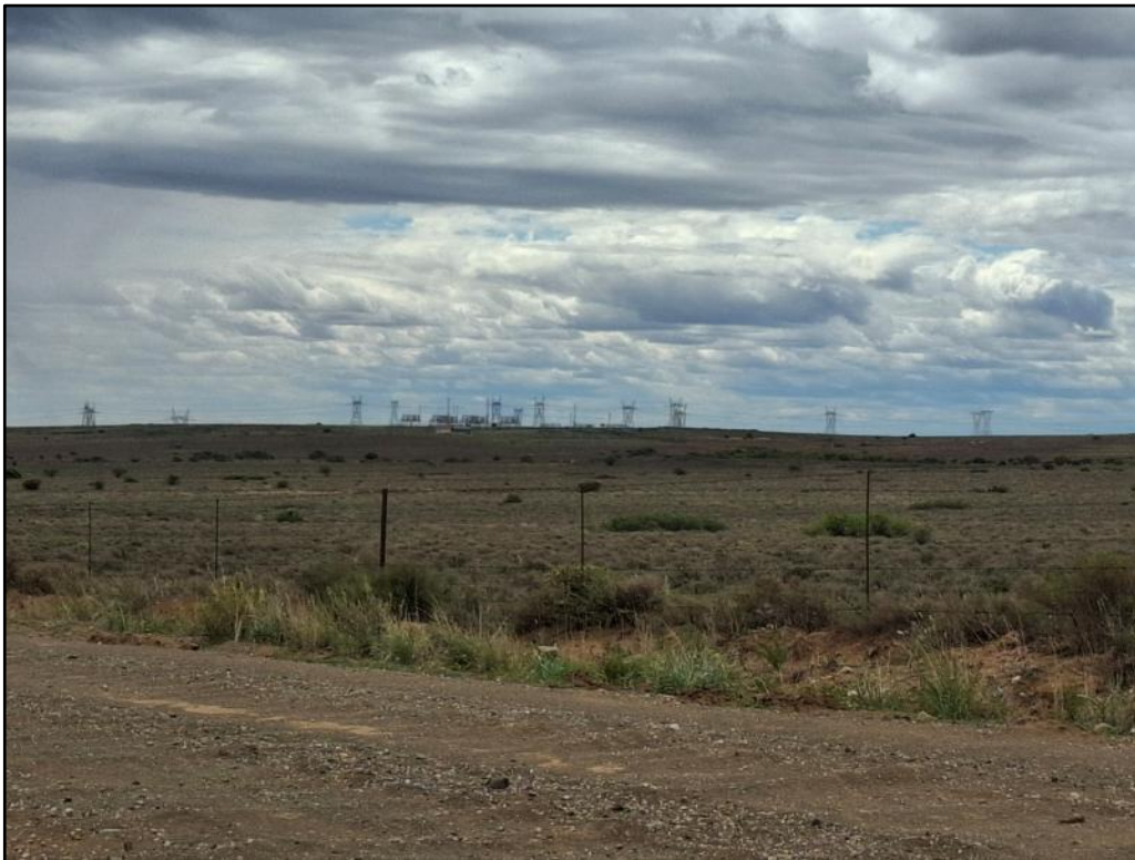
Photograph 3.5: Eskom substation north of S129
