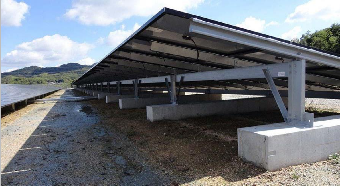
Figure 3: Cast Concrete Foundation - alternative mounting (Cape EAPrac, 2022)
