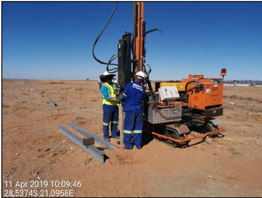
Figure 7: Ramming of steel piles into the pre-drilled / backfilled holes.
