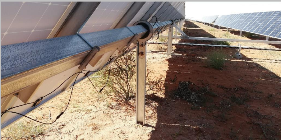
Figure 8: Completed ramming and assembly showing vegetation remaining intact beneath the modules.
