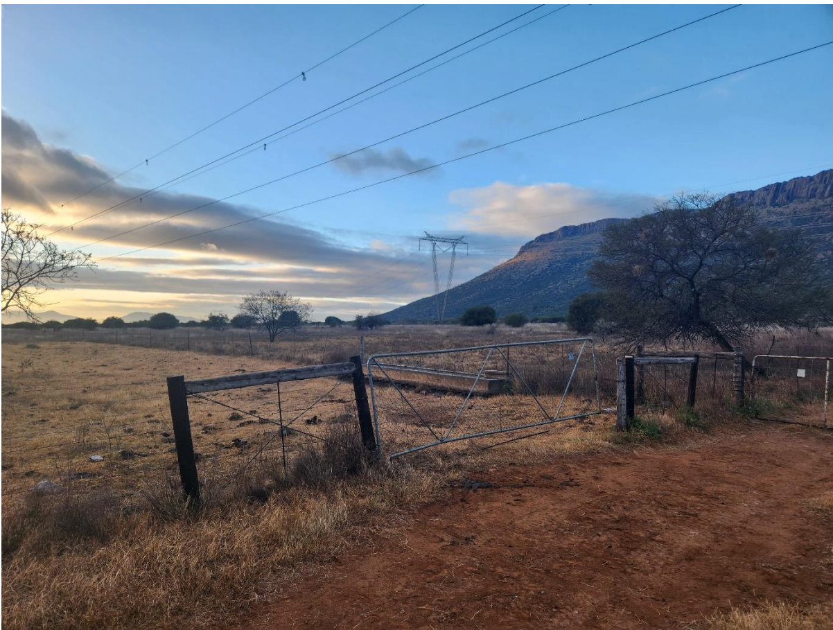
Figure 8: Eskom Existing 132kV and 400kV Powerline situated on the south of the Proposed PV Footprint.
