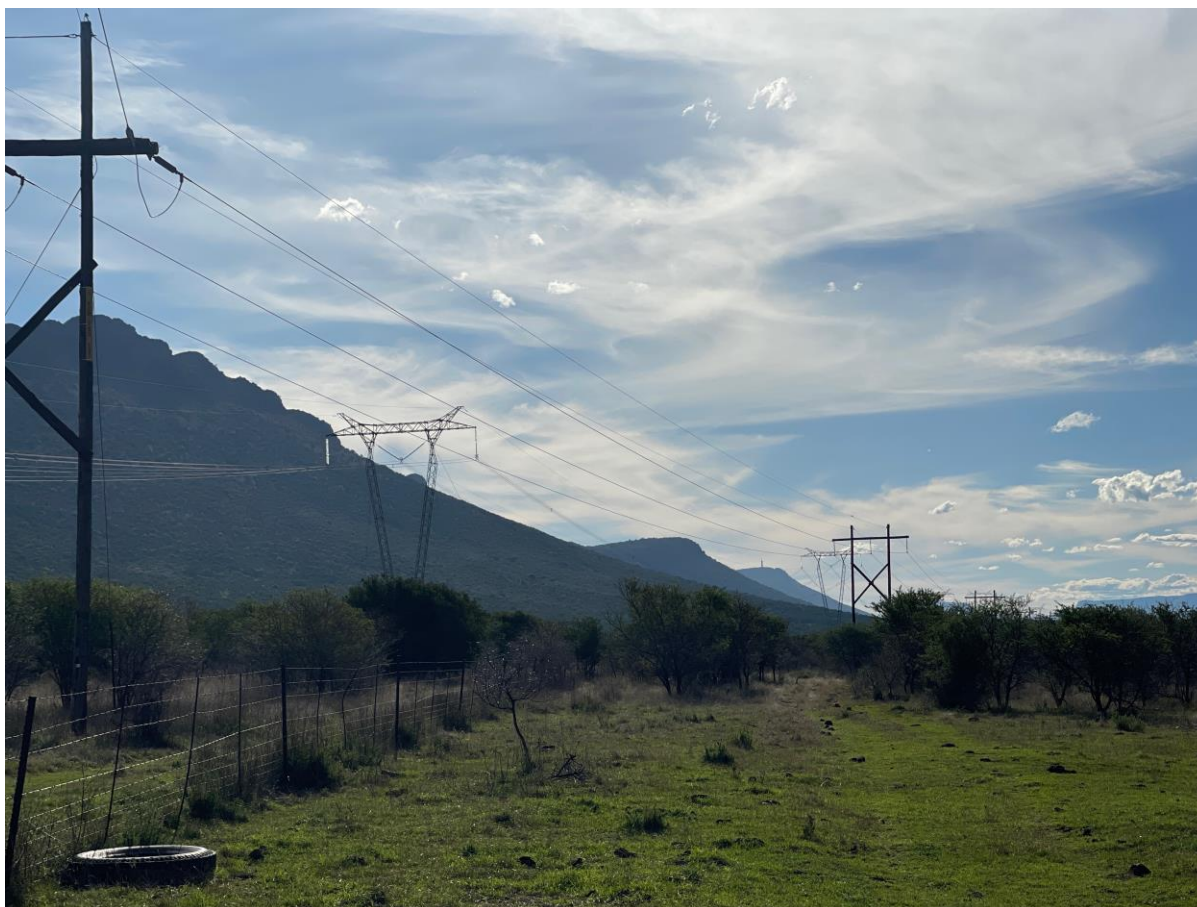
Figure 6-1 Negative impacts identified across the project area
