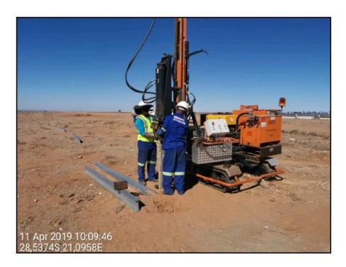
Figure 11: Ramming of steel piles into the predrilled / backfilled holes.
