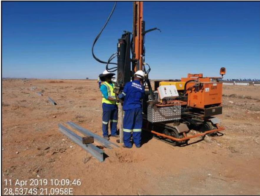
**Figure 11:** Ramming of steel piles into the pre-drilled / backfilled holes.
