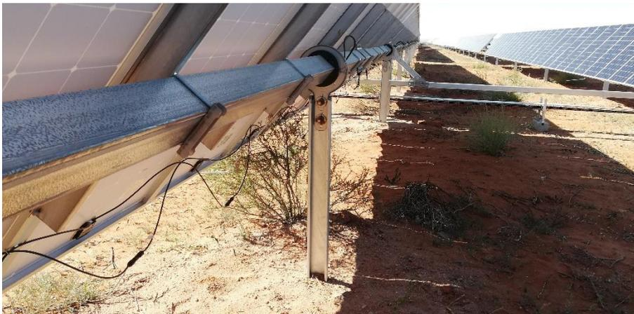
**Figure 12:** Completed ramming and assembly showing vegetation remaining intact beneath the modules.
