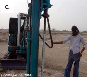
**Figure 8:** Mounting Structures. A) Cast Concrete Foundation. B) Driven/Rammed Steel Pile. C) Ground / Earth Screw Kareerand BESS (PV (Pty) Ltd)
