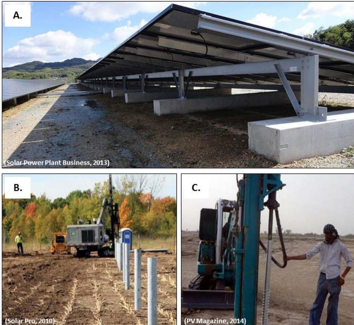
**Figure 8:** Mounting Structures. A) Cast Concrete Foundation. B) Driven/ Rammed Steel Pile. C) Ground / Earth Screw Kareerand BESS (PV (Pty) Ltd)
