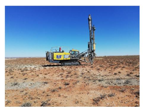
**Figure 9:** Predrilling of holes prior to the ramming of steel piles.
