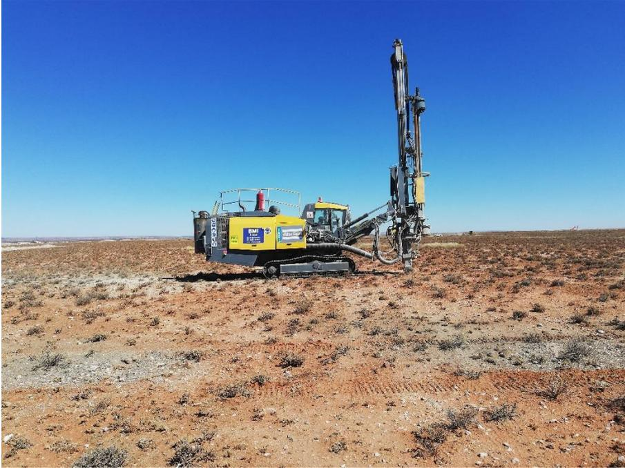
**Figure 9:** Pre-drilling of holes prior to the ramming of steel piles.
