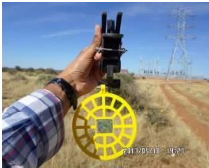
**Figure 24:** An example of a bird flight diverter to be used on the powerline: Viper live bird flapper.
