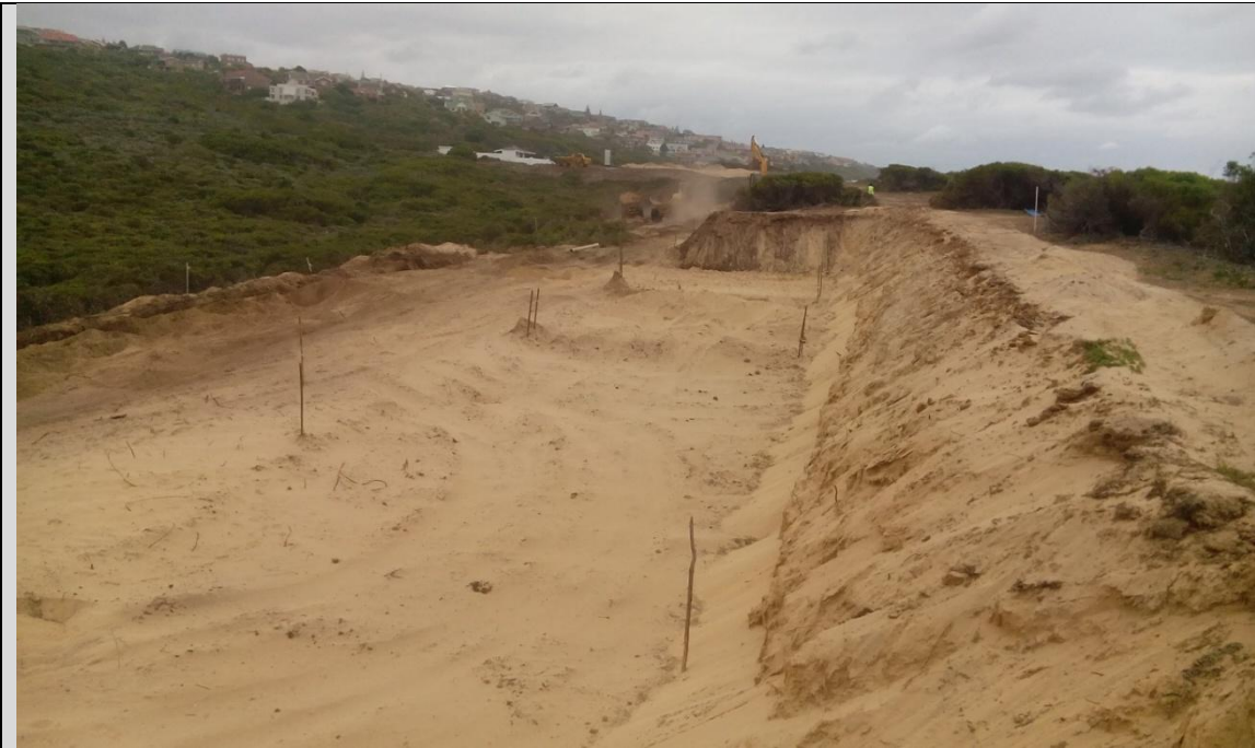
Figure 3: The building platform of the South Western apartment block was completed.
