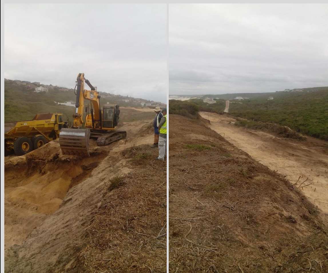
Figure 4: The full extent of the road was constructed.
