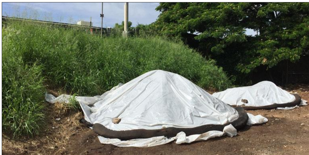
Figure 19. Stockpiles of fine textured building materials and soils covered with geotextile/plastic covering and banded with sandbags when not in use.
