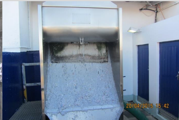
Photo 8: The mesh screen filtering discharge water from the offloading and processing activities
