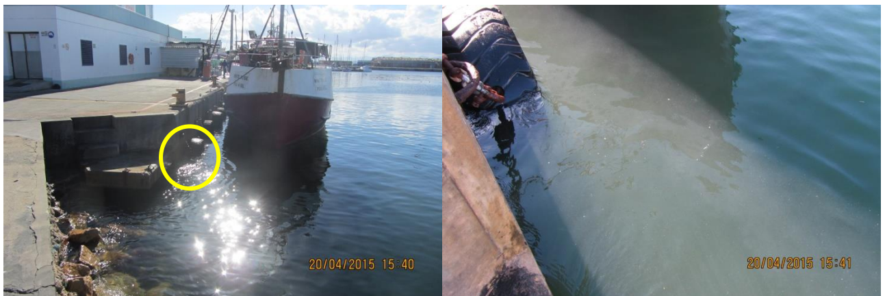
Photo 1: Discharge pipe is located at the steps
