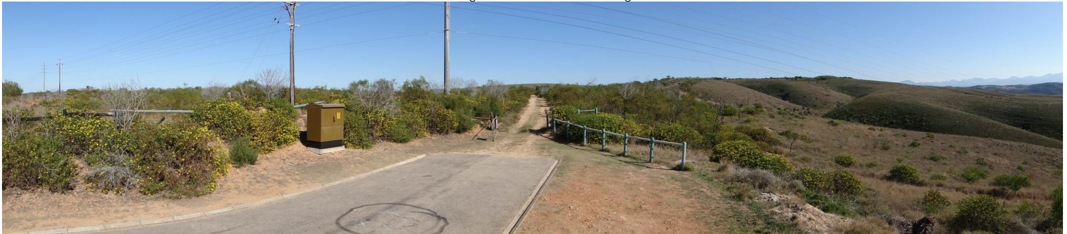
Photo 2: Main access onto the property from Geelhout Street.
