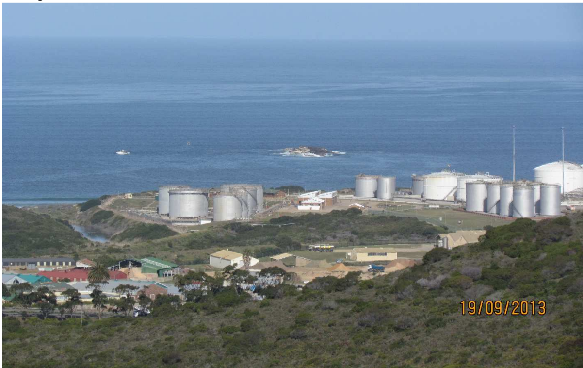
Oil Depot towards the South East
