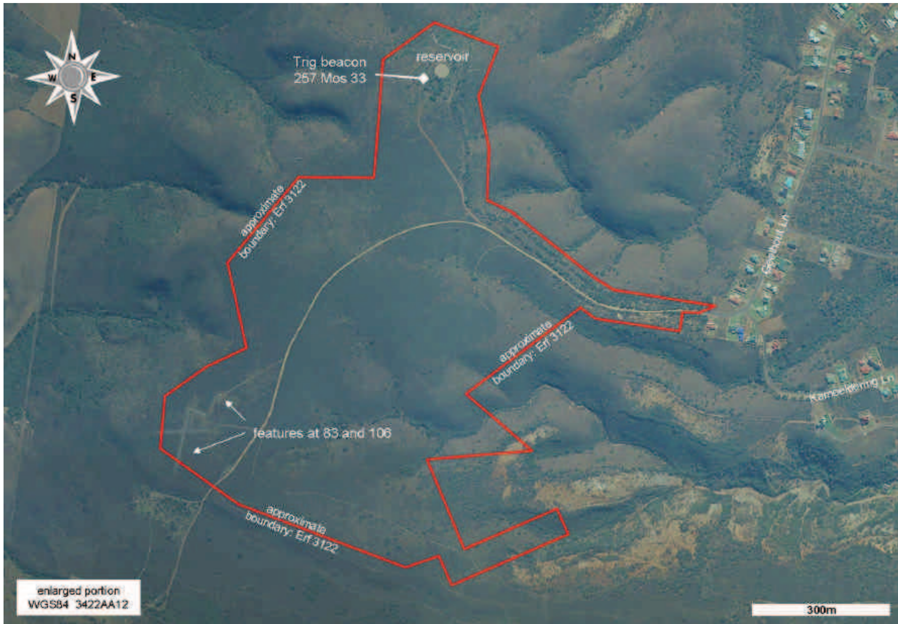
Figure 2. Enlarged area as indicated in Figure 1 showing property boundary & features. Courtesy of CDSM.
