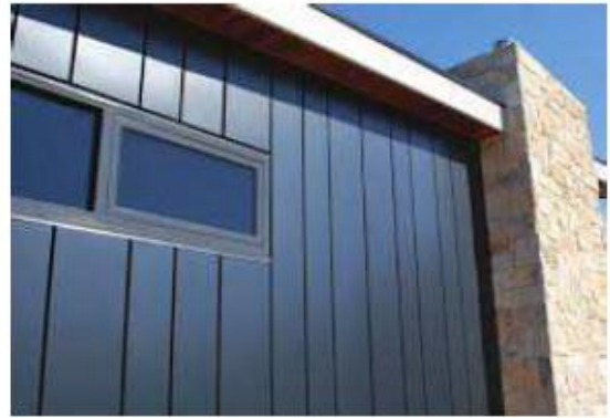
Figure 3 Typical sheet metal wall cladding
