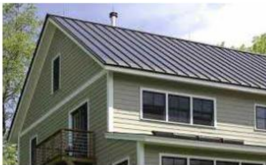
Figure 4 Typical klip-lok roof sheeting
