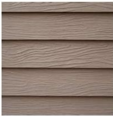
Figure 2 Typical fibre cement wall cladding
