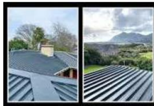
Figure 5 Typical IBR roof sheeting
