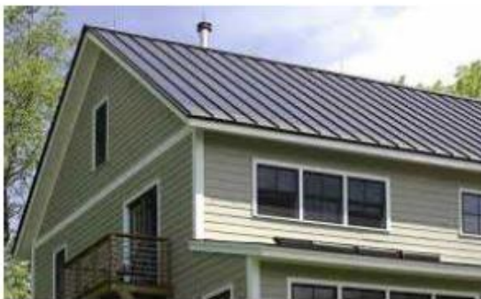
Figure 4 Typical klip-lok roof sheeting
