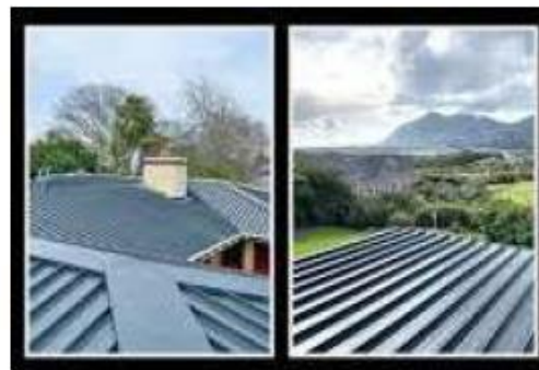
Figure 5 Typical IBR roof sheeting
