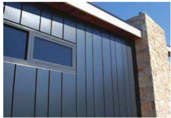
Figure 3 Typical sheet metal wall cladding
