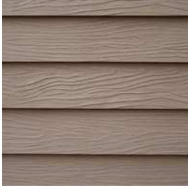
*Figure 2 Typical fibre cement wall cladding*
