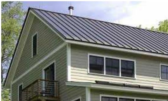
*Figure 4 Typical klip-lok roof sheeting*
