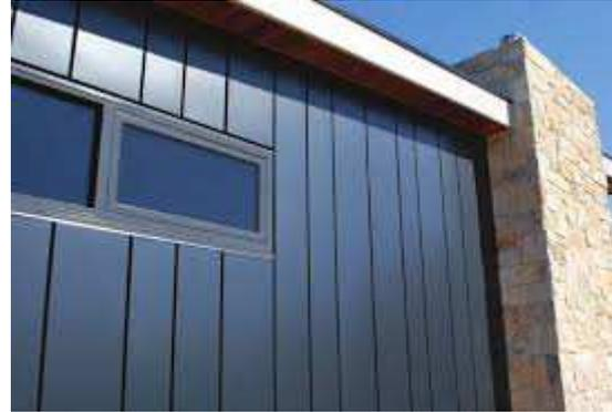
*Figure 3 Typical sheet metal wall cladding*
