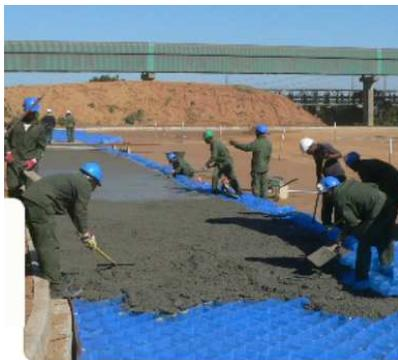
*Figure 10 Hyson Cells filled with concrete*
