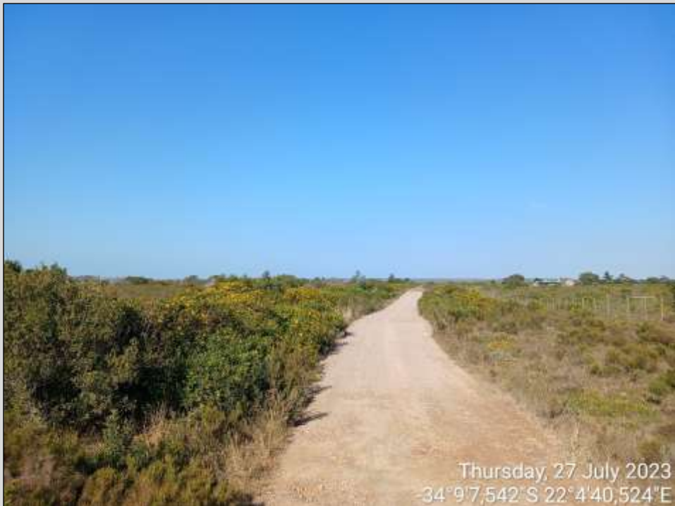
Figure 11: Photograph of existing Skilpad Street (west of 209/220).
