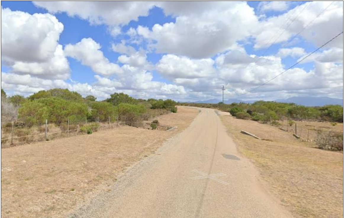
Figure 11: Culvert on eastern boundary underneath Klipheuwel Road.
