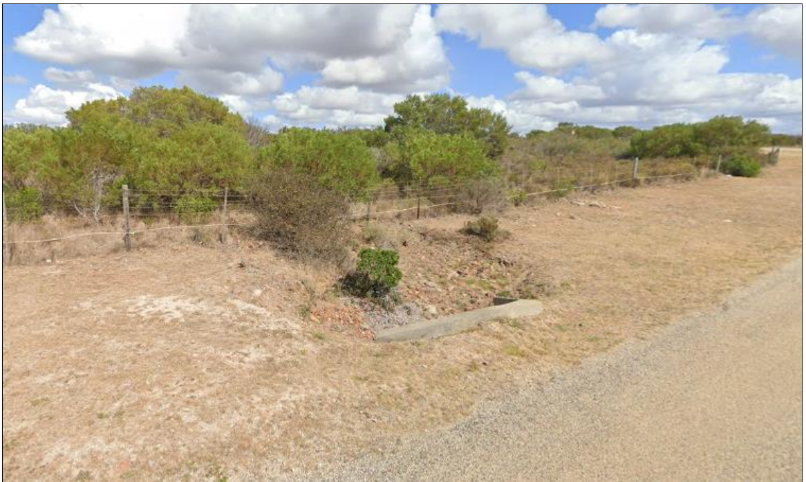
Figure 12: Culvert on eastern boundary underneath Klipheuwel Road.
