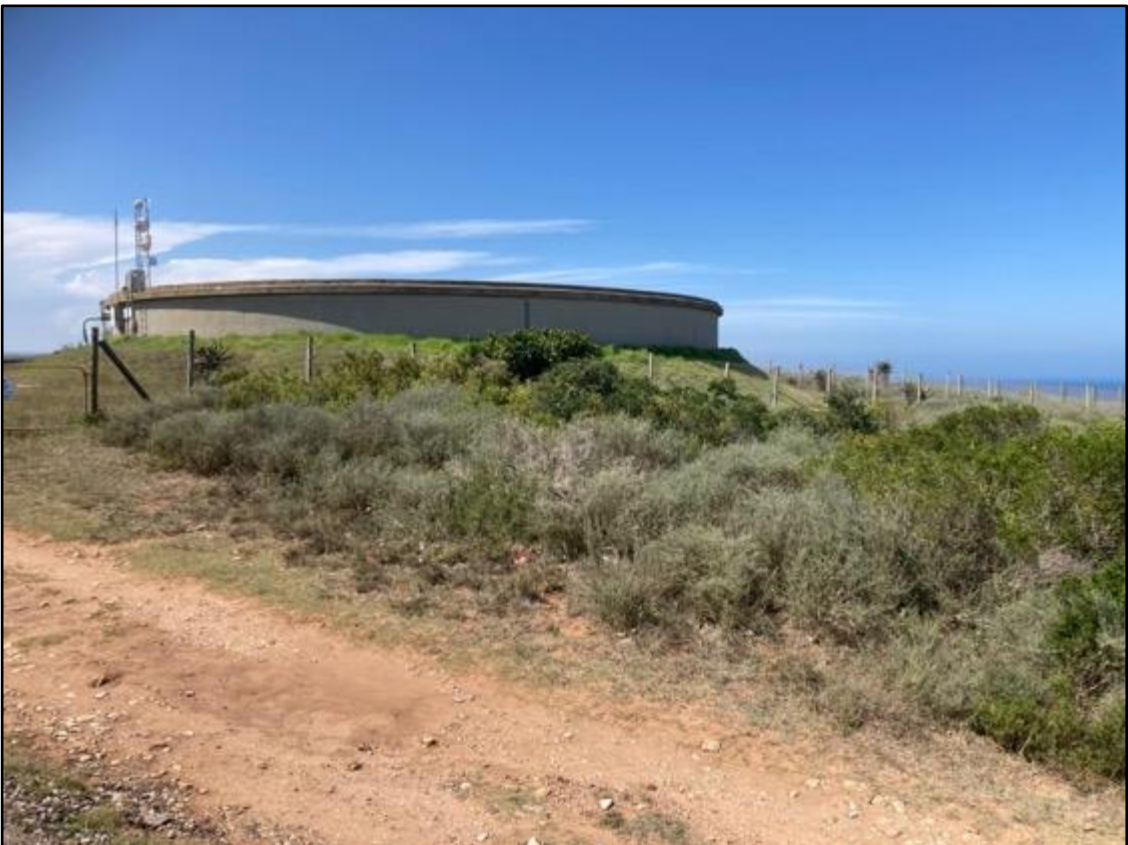
Figure 13: Reservoir in centre of site.
