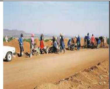
Dirt road build wit Hyson Cells. No-concrete
