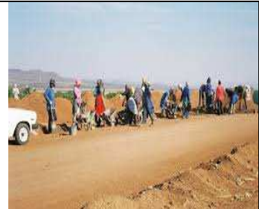
Dirt road build wit Hyson Cells. No-concrete
