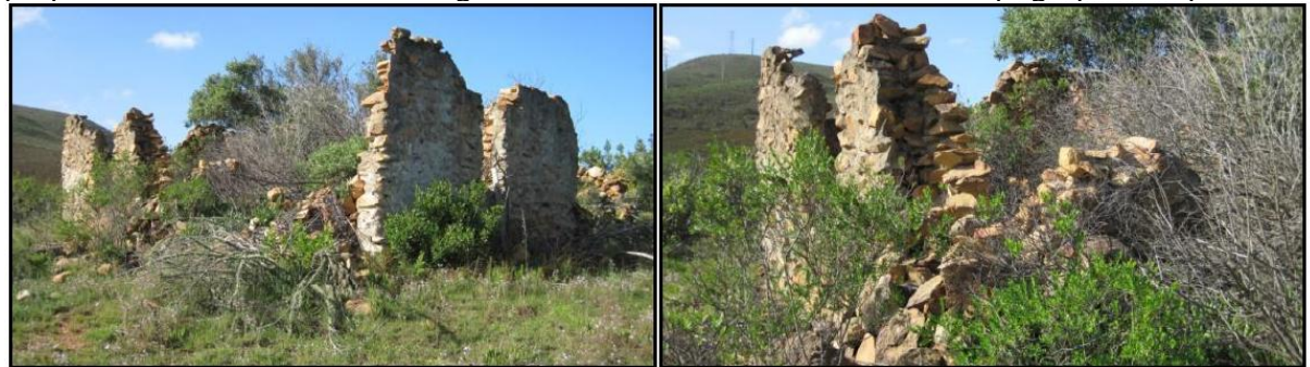
Figure 43: Remnants of an old building (Source: HIA, 2024).
