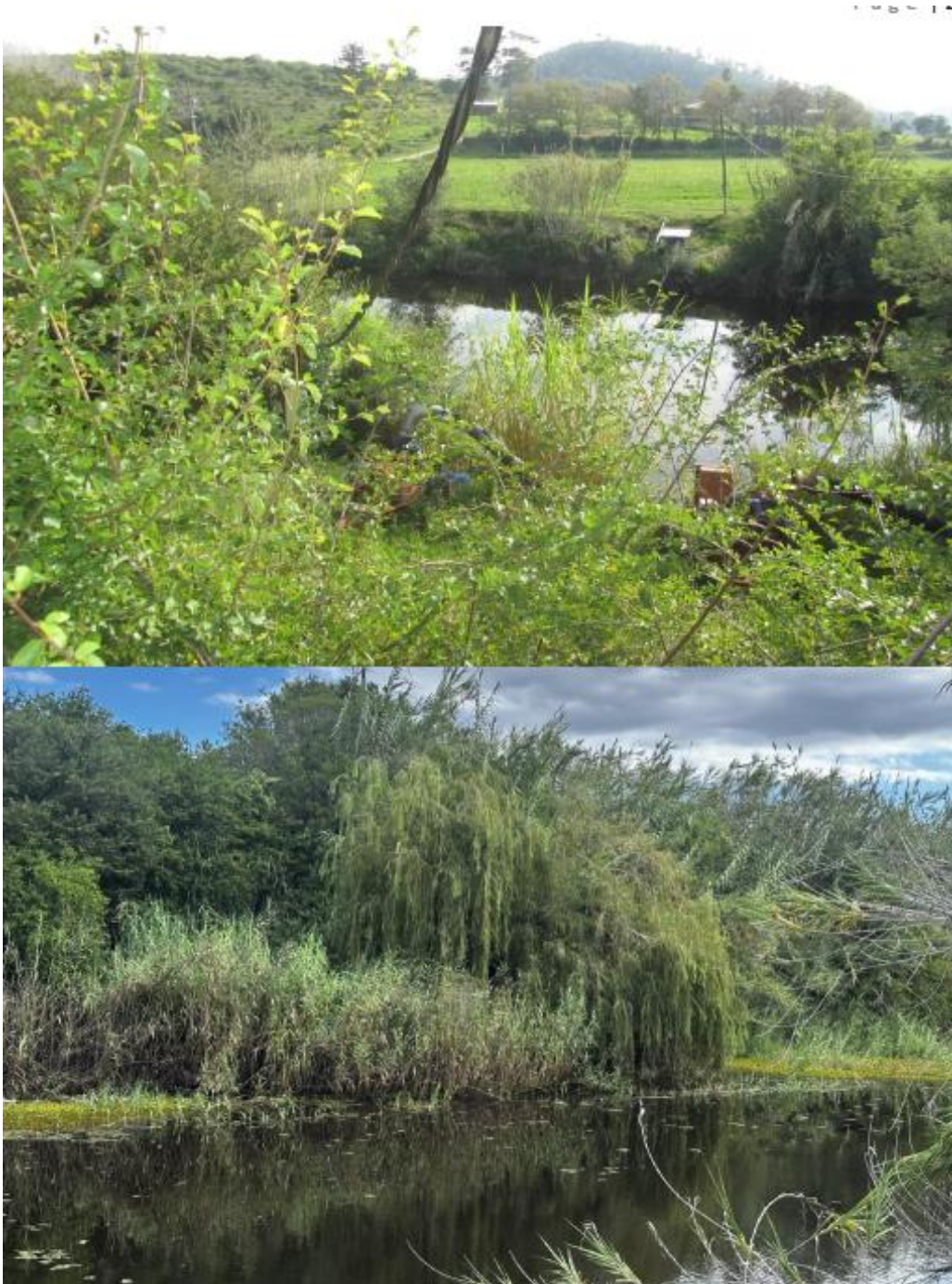
Figure 27: Existing abstraction point for the farm's irrigation supply (Source: BlueScience, 2026).
