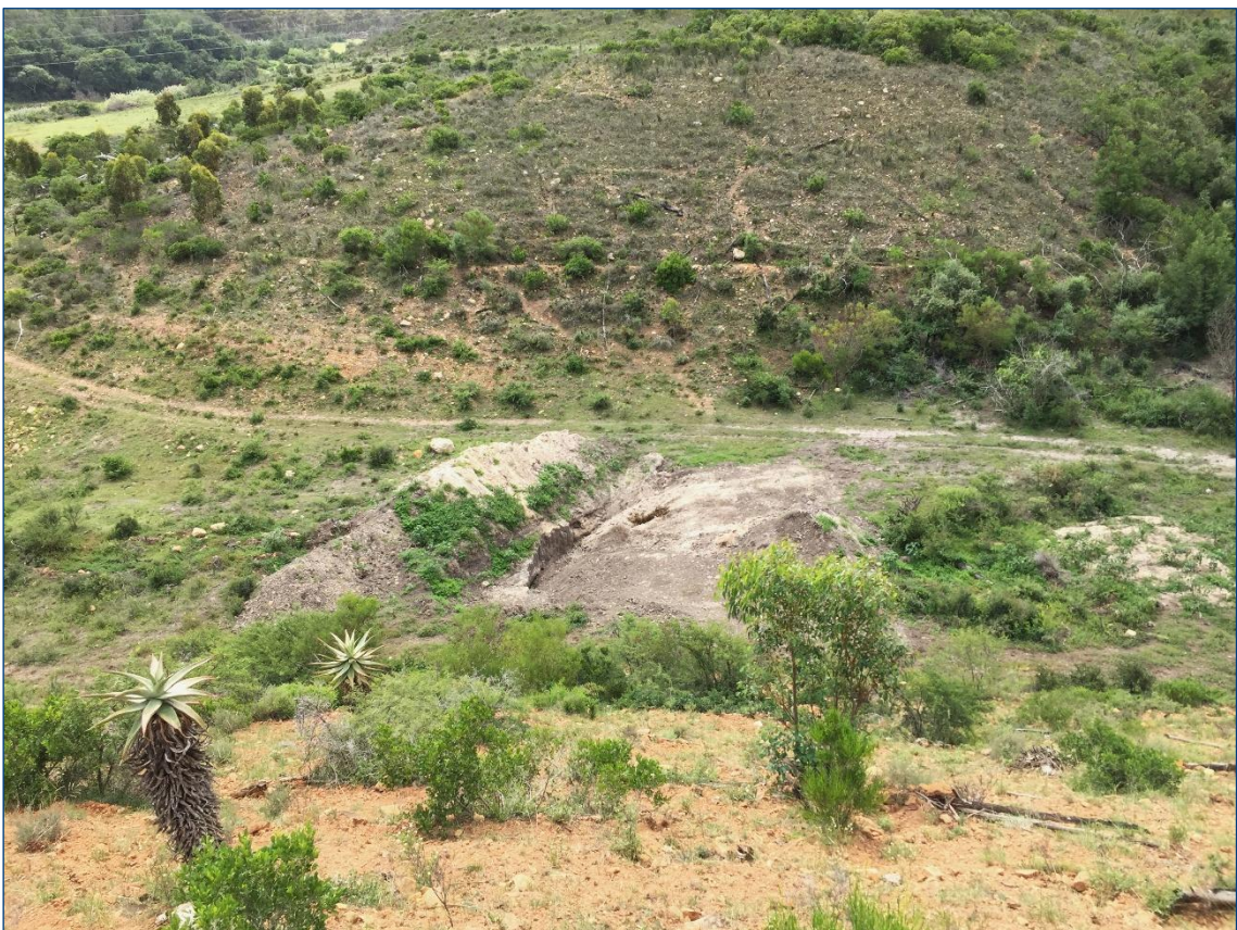
Figure 5-5: Degraded lower end of site and position of the proposed dam wall.
